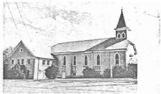
The building after 1953
